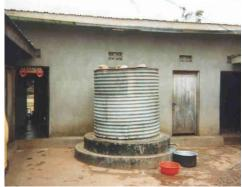
Figure 4b: A corrugated iron RWH tank in Uganda
