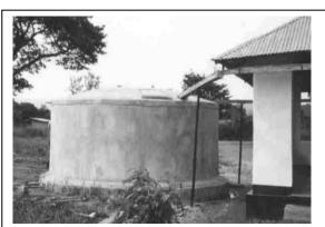
**Figure 5 :** Ferrocement tank in Ruganzu Village, Tanzania. Photo credit: DTU
