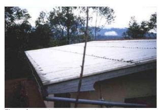
**Figure 1:** A typical corrugated iron sheet roof, showing guttering. Photo: Practical Action
