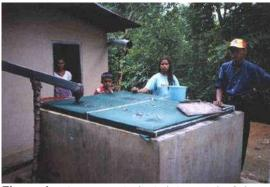
Figure 4a: An owner-built brick tank in Sri Lanka
